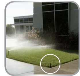
Spray body with broken nozzle with x-Flow
